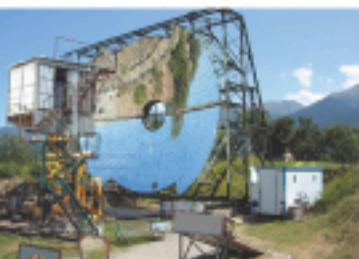
The solar furnace in Mont Louis, built in 1949 by Professor Félix Trombe, was the first solar furnace in the world. This dual reflection solar furnace has been in steady evolution over the past 50 years and in
